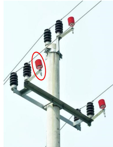
Fig. 11 A 10 kV transmission line with compressing arc extinguishing device in Guangxi, China
