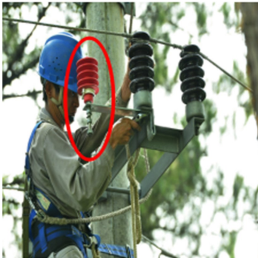
Fig. 1 On-site installation picture of compressing arc-extinguishing device
