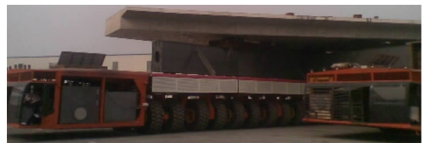
(a) Single vehicle with bridge driving on the cross-slope
